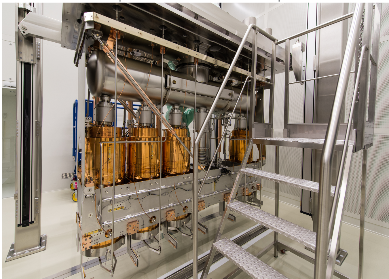
Header Image: HIE-ISOLDE infrastructure. (Image: CERN)
